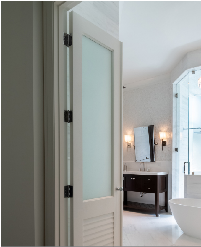
Flat Jambs with Applied Stop
